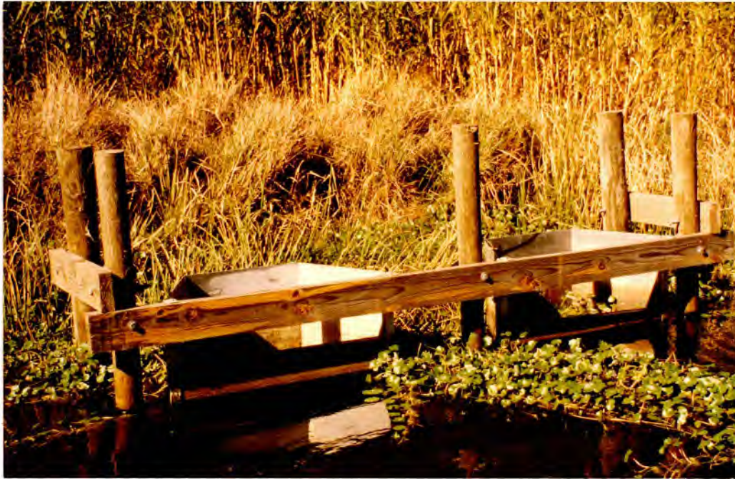
FIGURE 1 Stoplog water control structure, J.D. Murphree Wildlife Management Area, Texas.
