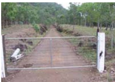
In places along the Moore–Linville section (such as north of the old transfer station), the gravelly ballast material was mixed with excavation spoil (obtained from a creek crossing), graded and rolled to provide the finished surface.
