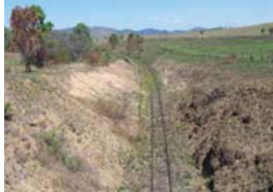
Above: The formation travels through typical rural countryside in large cuttings and on top of embankments
