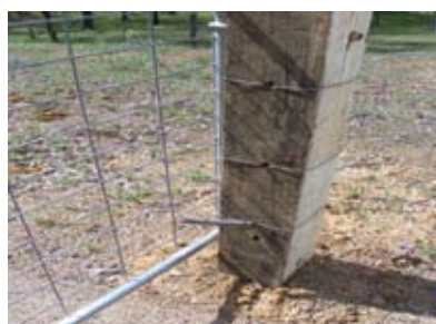
Self-closing gates (as installed on the Moore–Linville section) should prevent livestock from wandering away from any land leased to adjoining landholders.
