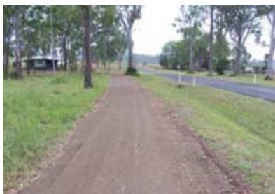
On the new trail section immediately north of Moore, a layer of crusher dust was placed over the existing base soil. This material source was sedimentary in nature—Esk Shire Council (the contractor) believes it will perform similarly to the material on the existing Fernvale–Lowood section of the trail.
