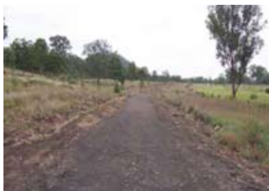
A number of sections were found to have ballast that was reasonably fine. Esk Shire Council engineers decided to leave the surface as it was (no additives) to see how it performed, so these sections were reworked to give a smooth surface. Most of this material appears to have a high proportion of waste ash. This material is less cohesive than other sections. If it deteriorates under use in the trial section, it will be overtopped with crusher dust. This section is immediately north of the Moore Cemetery.
