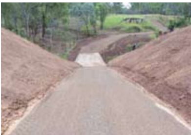
Above: All bridges in this section have been removed. The new work has involved the development of a graded entry with a concrete floodway at the base. This is the work at Boundary Creek.
