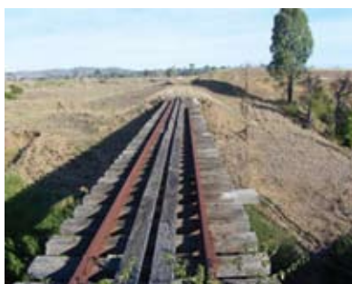
The Lillydale to Warburton Rail Trail provides for all users, including horses. Some of the bridges are more than 5 m above the ground. Appropriate handrail heights ensure safety for all users. Similar handrails should be provided on high bridges along the Brisbane Valley Rail Trail, such as this one at Jimmy’s Gully.
