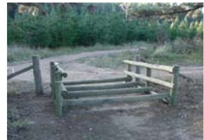
Feedback from horse riders indicated that the chicane gate was difficult to manoeuvre horses through (although it is understood that there have not been difficulties on the Lilydale–Warburton Rail Trail). One of the issues was getting the dimensions of openings exactly right. Consequently, both narrower chicanes (bike and pedestrian only) and cavaletti gates at all major and remote road crossings are now recommended.
