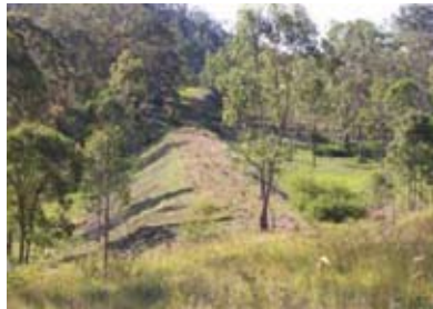
Above: Embankments will be a feature of the rail trail—this embankment, just north of the Brisbane Valley Highway overpass, is amongst the highest along the corridor
