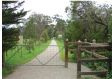
Gates/chicanes on the Lilydale–Warburton Rail Trail are effective in allowing legitimate trail users, and excluding unwanted and unwelcome users such as motorcyclists. A similar gate was installed on the Moore–Linville section near the Moore Cemetery.
