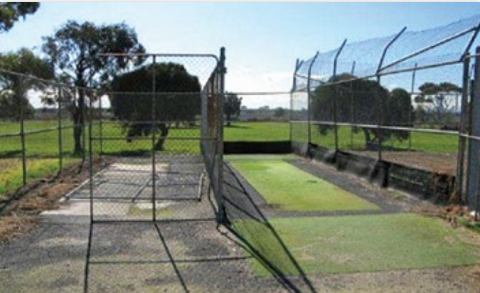
Infill previous safety and maintenance hazard area with compacted granitic sand and 25mm pile synthetic grass.
