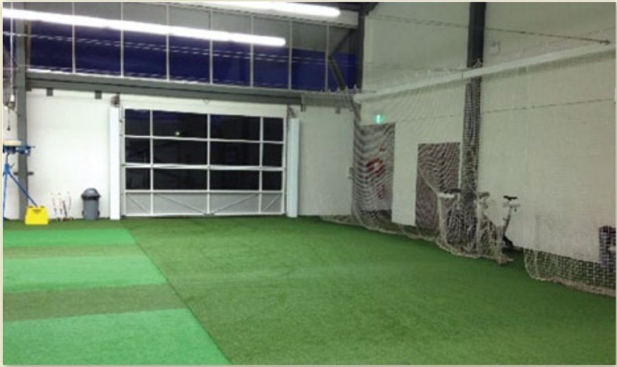
Roller door Roller door opens up to the main playing field and spectator concourse and promotes multi-use options and creates better airflow and ventilation during summer months.
