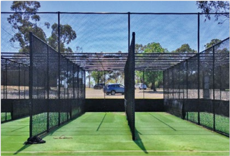
The adjacent image provides an example of the Australian Standard 9m netting roof length. It also demonstrates a design option for minimising the impacts of errant balls travelling over the roof of the net and damaging neighbouring property and/or passers by.
