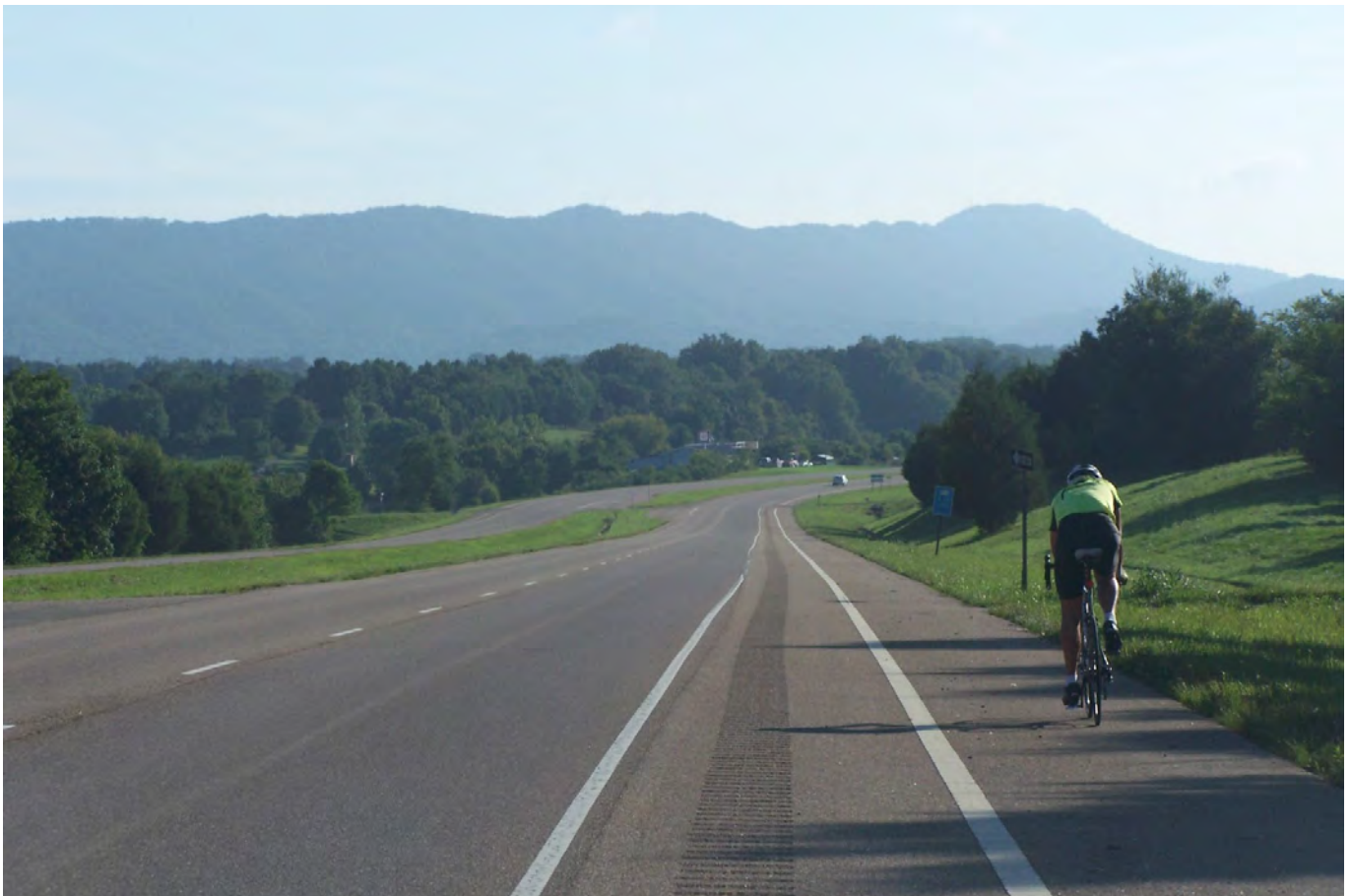
EXAMPLE OF WIDE ROAD SHOULDER AND 'VIBRA-LINE'
