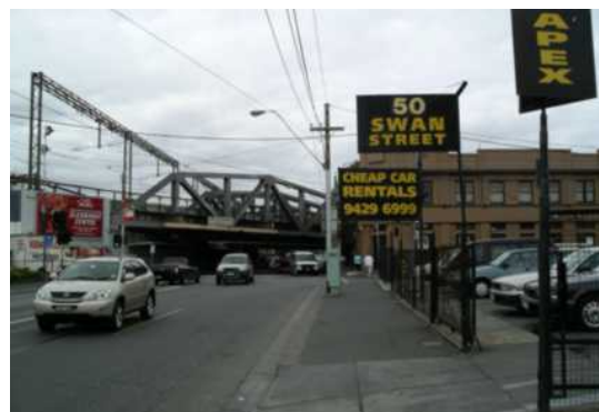
Figure 28 Pedestrian access to Swan Street shops is under the railway bridge
