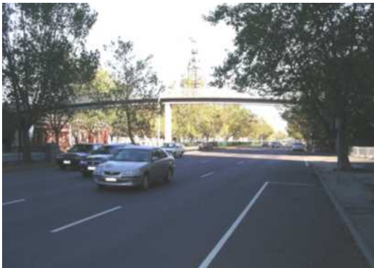
Figure 11 Hoddle Street looking south and the Vere Street overpass
