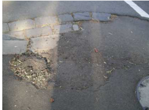
Figure 24 Surface break-up, Alexandra Parade
