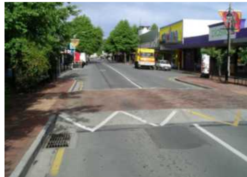
Figure 26 A raised pedestrian crossing, in a mid-block location, Nelson, New Zealand
