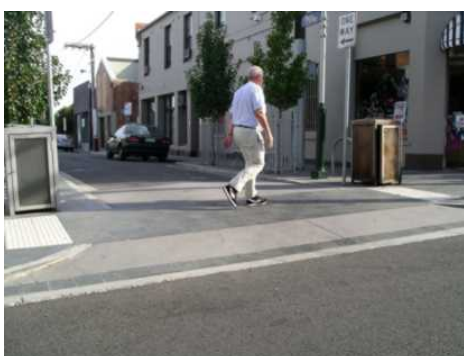
Figure 26 A raised pedestrian crossing - Toorak Road, South Yarra
