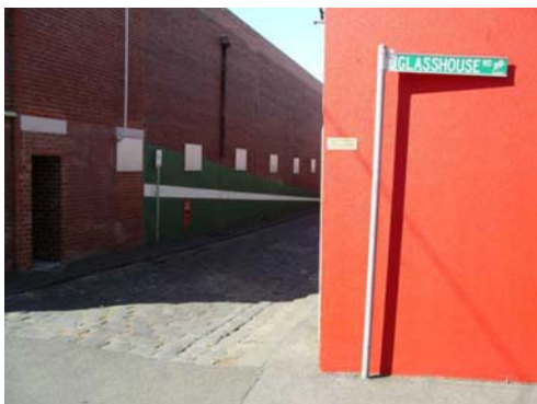
Figure 9 This sign has been installed at 90 degrees from the correct angle and thus mis-identifies the street
