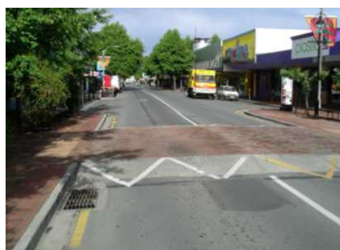
Figure 27 A raised pedestrian crossing, in a mid-block location, Nelson, New Zealand
