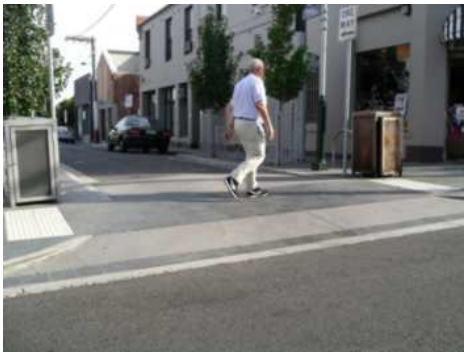
Figure 25 A raised pedestrian crossing - Toorak Road, South Yarra
