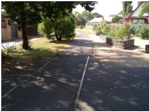
Figure 21 Shared path adjacent to North Fitzroy primary School on Fergie Road
