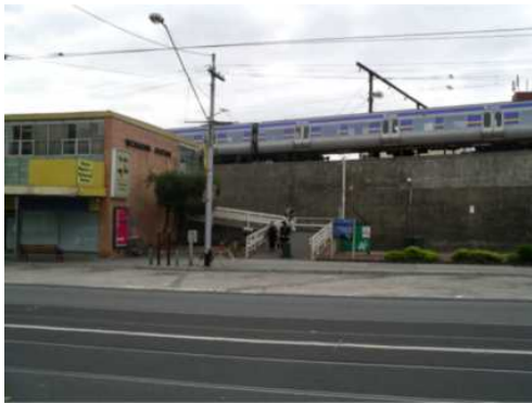
Figure 27 The South entrance to Richmond Station on Swan Street
