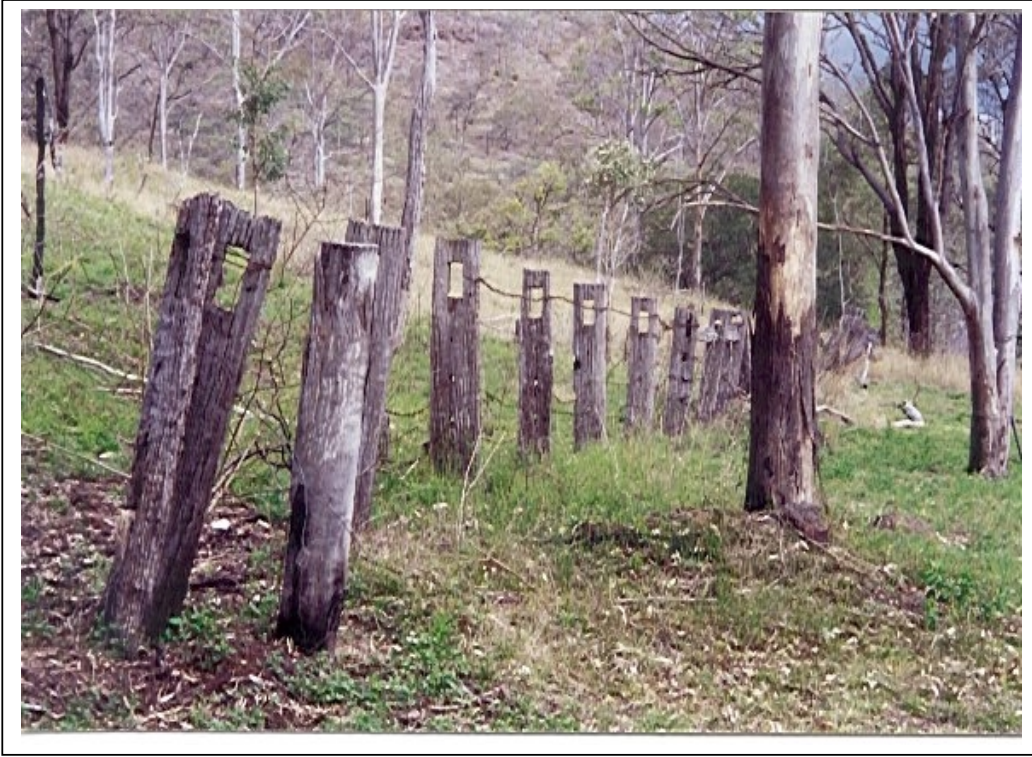
Glen Rock Place No. 18 - Square Post and Rail and Three Wire Fence (18.8.2000)
