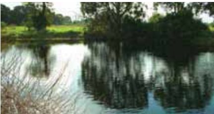
CONSTRUCTED DAM CLOSE TO MORDIALLOC SETTLEMENT CREEK
