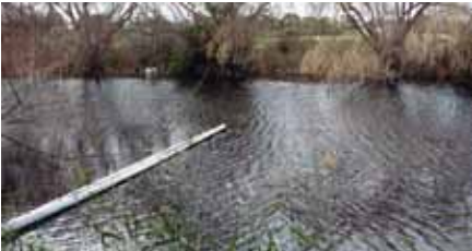
CONSTRUCTED DAM CLOSE TO MORDIALLOC SETTLEMENT CREEK
