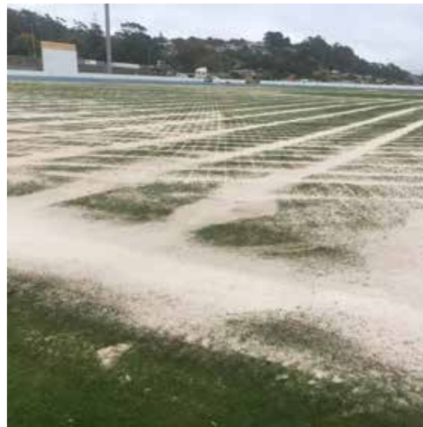
Installing sand slit drains into existing sportsfield
