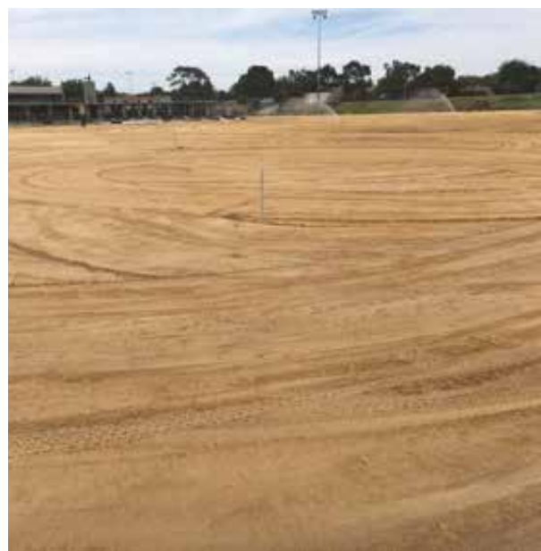
Installation of sand root zone layer
