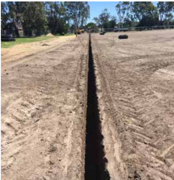
Trench dug prior to installing drain
