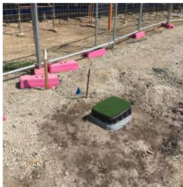
Installed solenoid box
