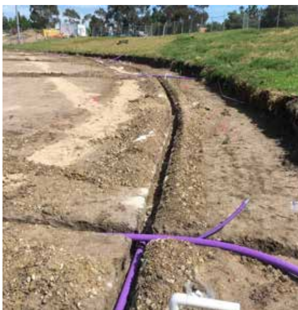
Installation of irrigation pipework
