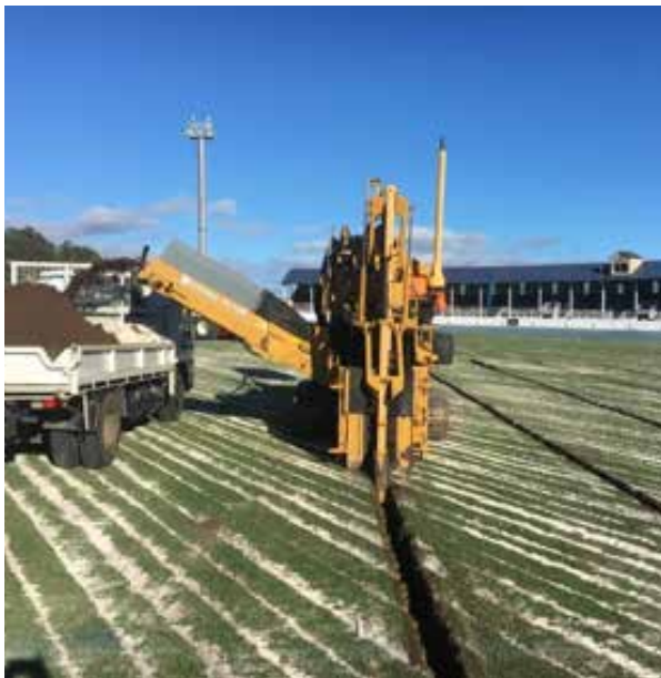
Installing sand slit drains into existing sportsfield
