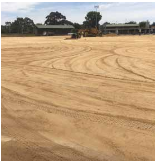
Installation of sand root zone layer
