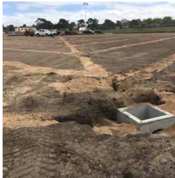
Subsurface drainage being installed in oval
