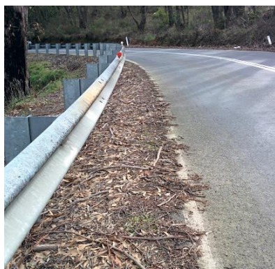
Figure 16: Cyclists are forced to use the traffic lane when shoulders are covered in leaf litter
