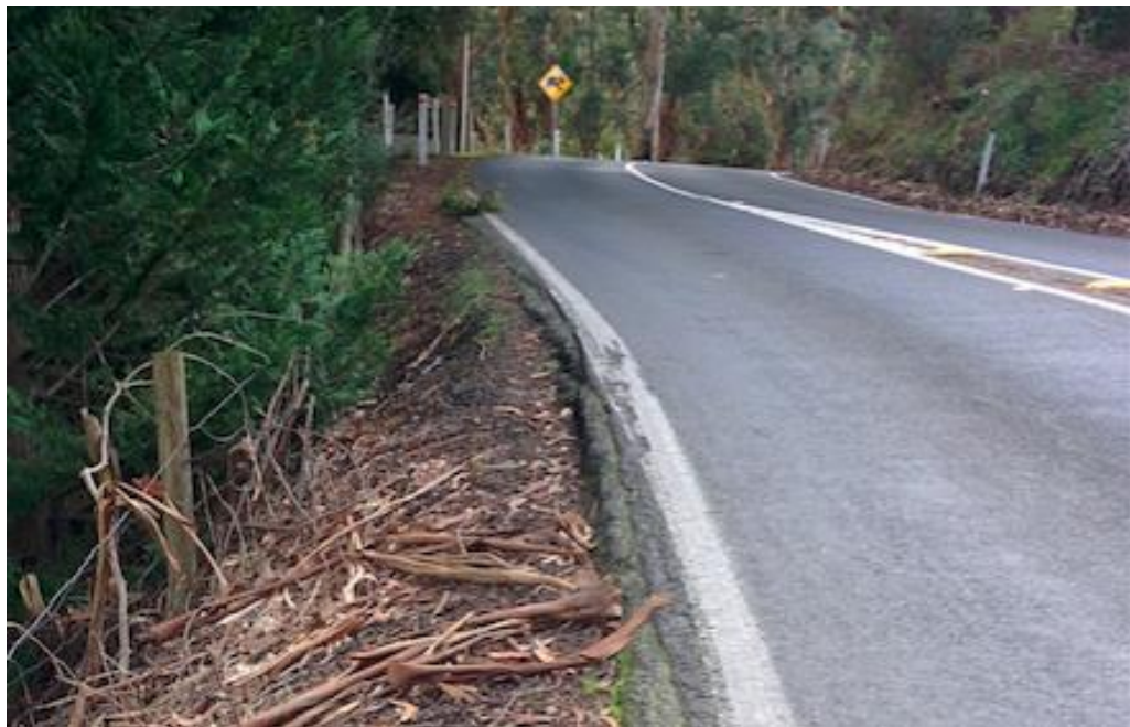
Figure 6: Sharp drop-off such as this are dangerous for cyclists who move over to let a car pass
