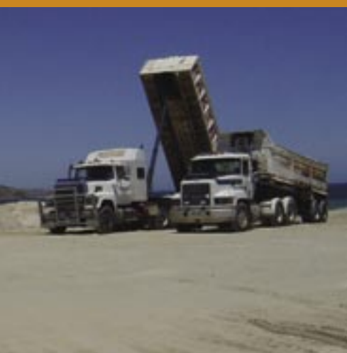
Sand dumping platform at Edwards Street, Brighton – trucks dumping sand on the platform
