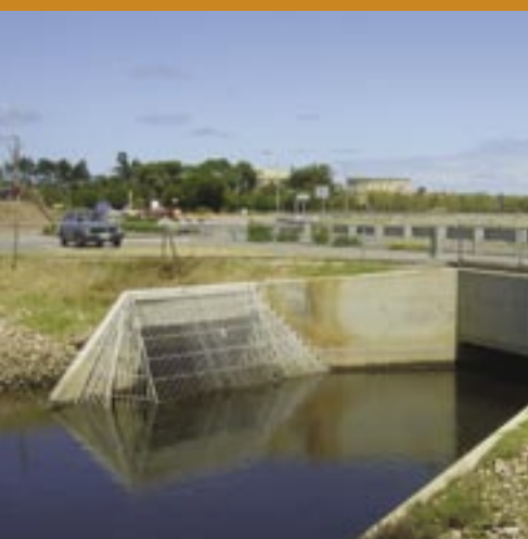
Trash rack covering Patawalonga Creek and Airport Drain into the Barcoo Outlet pipeline
