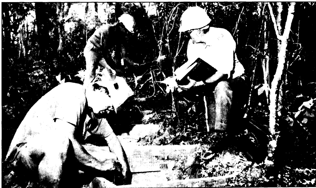
Path construction in Croajingolong National Park.
